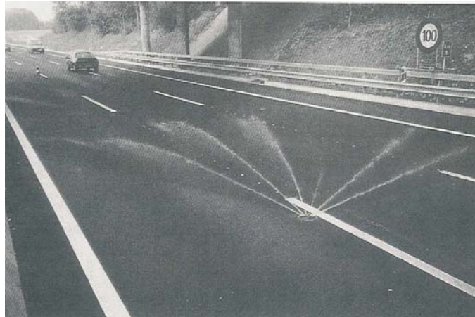
Figure 5: Spray head in action, automated salt spraying system in Lausanne, Switzerland.
